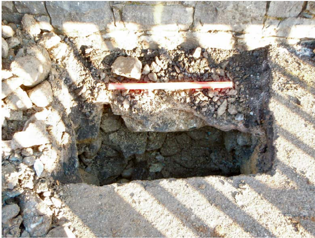
Plate 3: Site A, High Hill Wall. A north-facing view of HDP03, showing stone rubble footing for the adjacent flood wall
